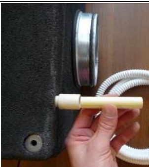
Connecting a straight condensate drain with a sleeve to connect the line
