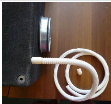
Inserting the line and securing it with a clip (the clip and the line is provided by the plumbing installation company)
