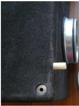
A condensate drain outlet from the door in section i 2 , with condensate drain accessories
