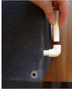
Connecting the condensate drain with a 90° elbow and connecting the line
